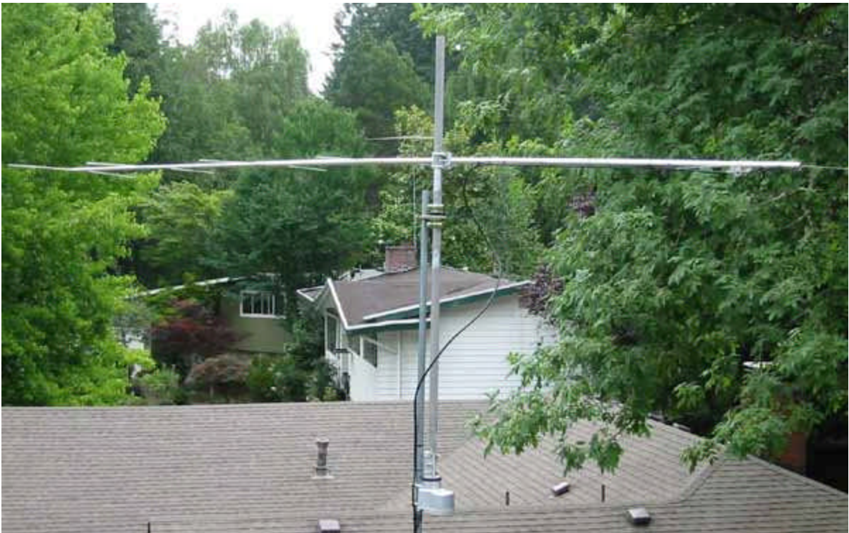
The rotor is bolted to the top 1.25 inch OD piece of the push up mast while the 1.5 inch OD rotating mast sits on top of the rotor. The bottom of the loop of transmission line (a 50 foot piece of LMR-400 with N connectors) is held to the fixed mast with cable ties.
